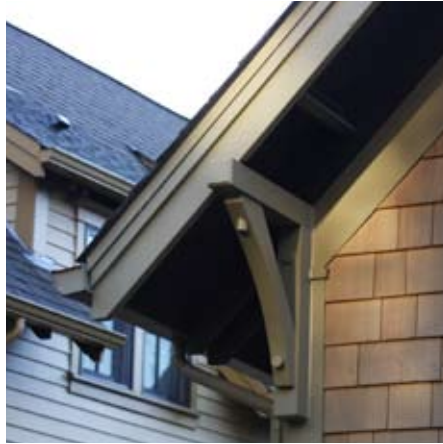
Open eave and bracket detail
